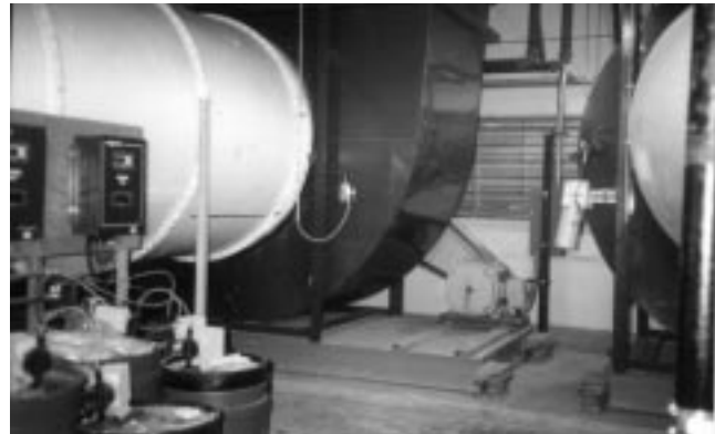
Figure 5. Fan mounted on an inertia base
