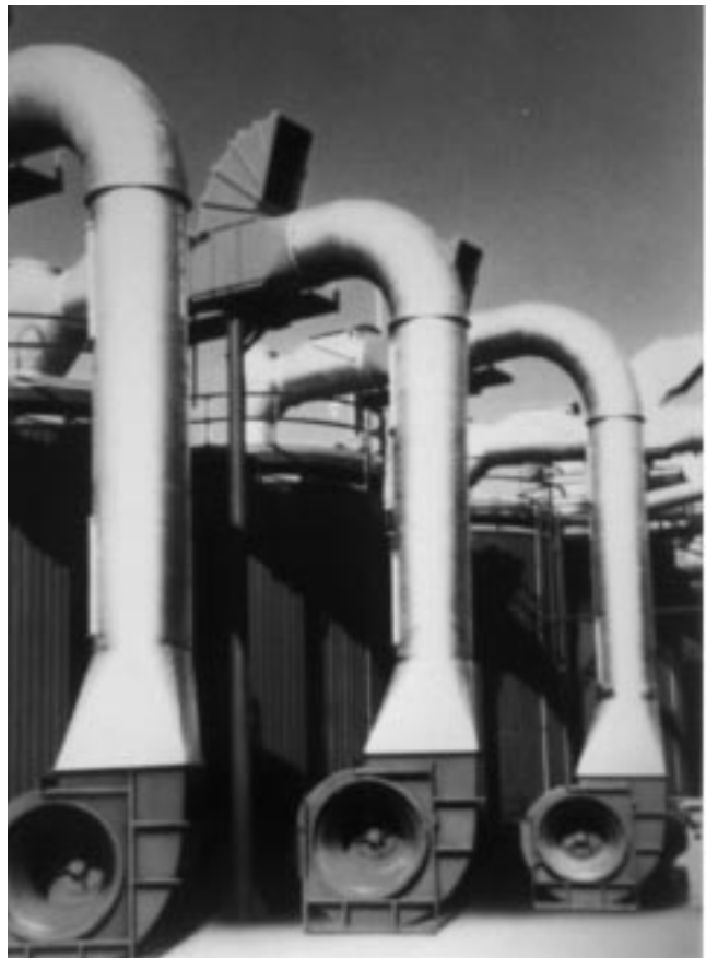
Figure 6. Well-designed duct configuration
